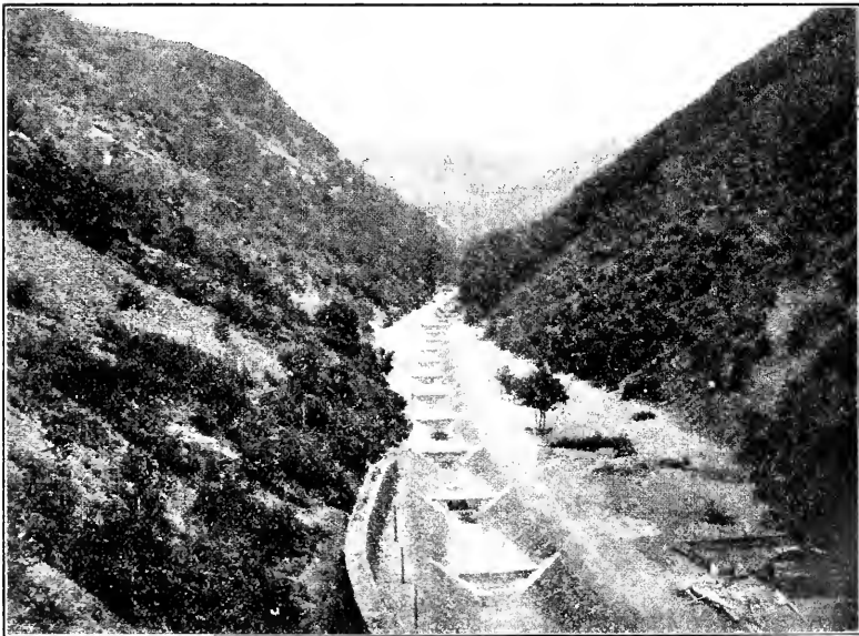
FIG. 2.—TYPICAL EXAMPLE OF WORK OF REFORESTATION AND MOUNTAIN-TORRENT CONTROL ON HEAD-WATERS OF ELBE RIVER.
